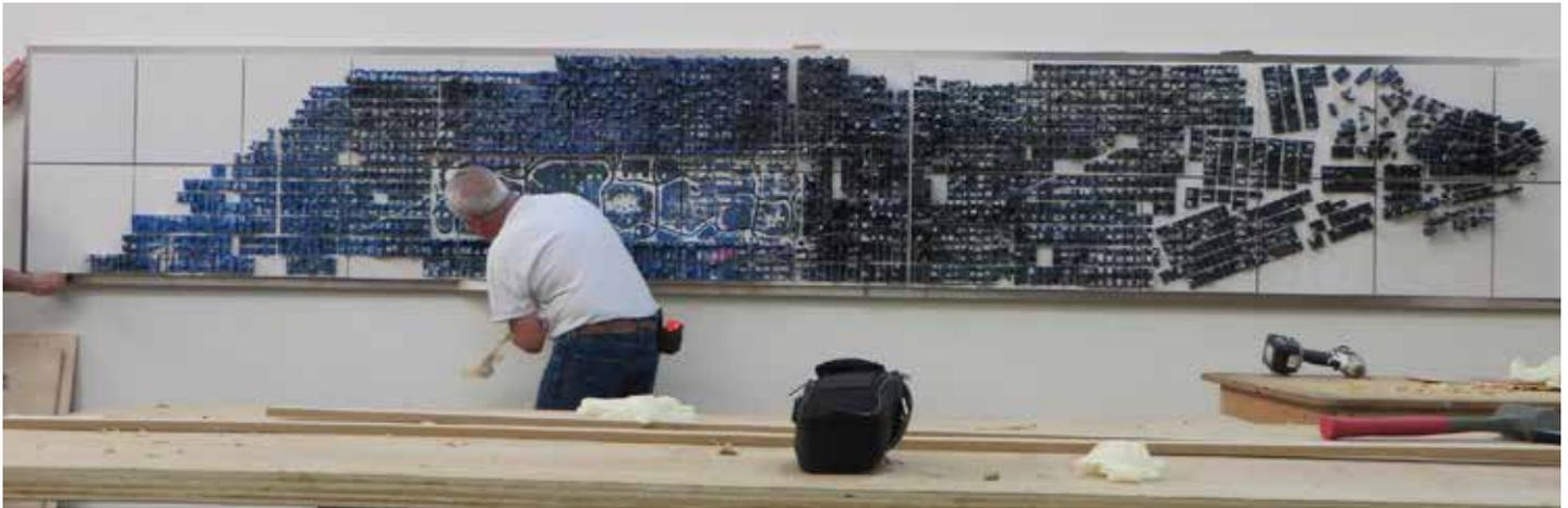
The project was not without its challenges. Considerable time was spent defining how the CAD software exported the data so it would work perfectly with the color jet printers. Another challenge involved engineering a way to permanently hang the 28 models onto a wall to create the expanse of Manhattan without fasteners being visible.
